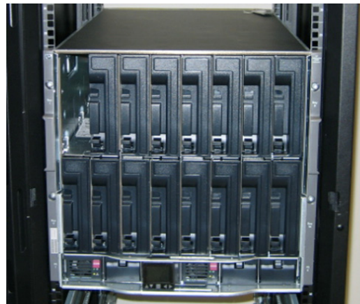
Figure 7B: The HP chassis installed on the rails.
