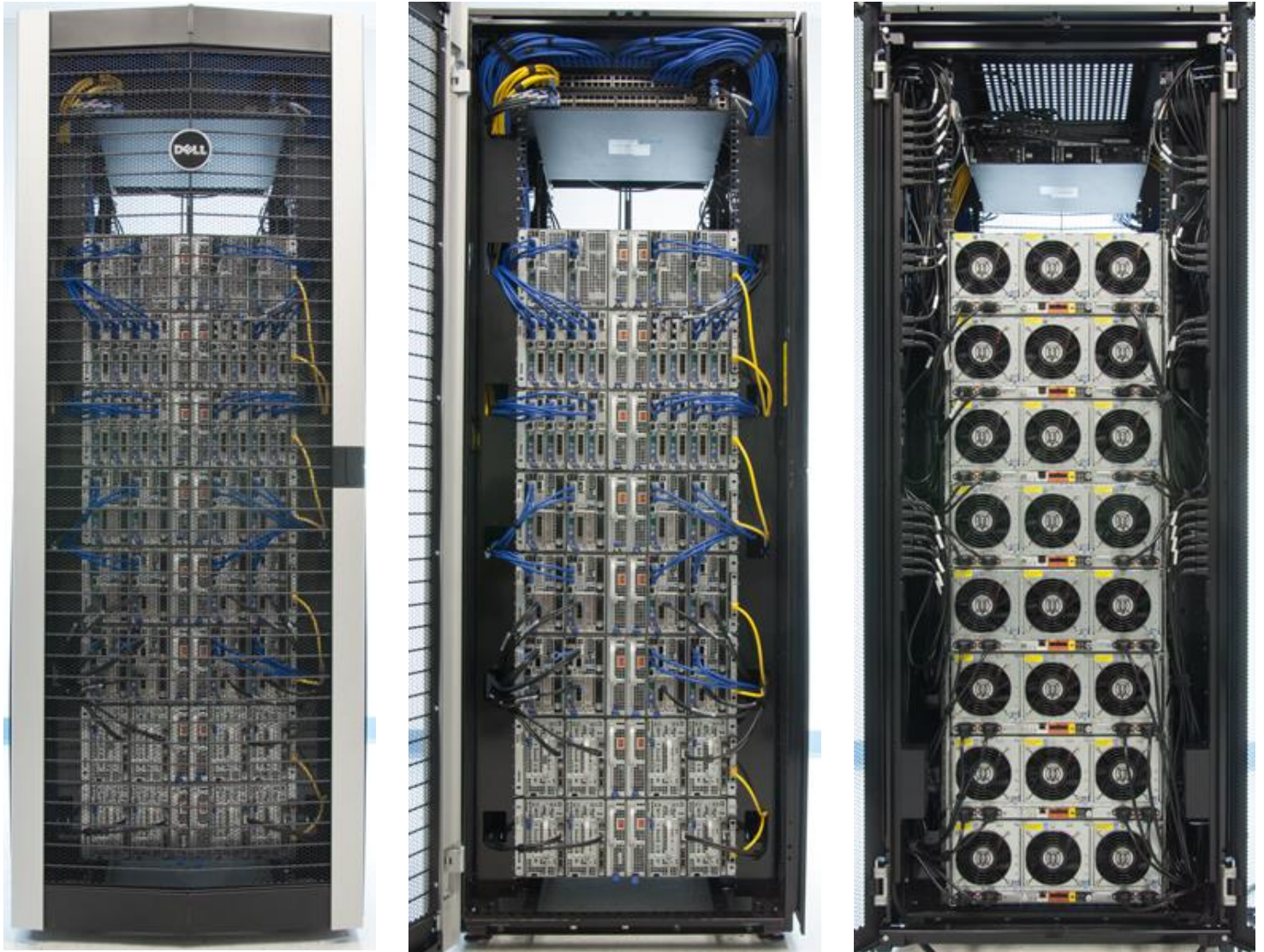
Figure 15: Three views of the completed installation.
