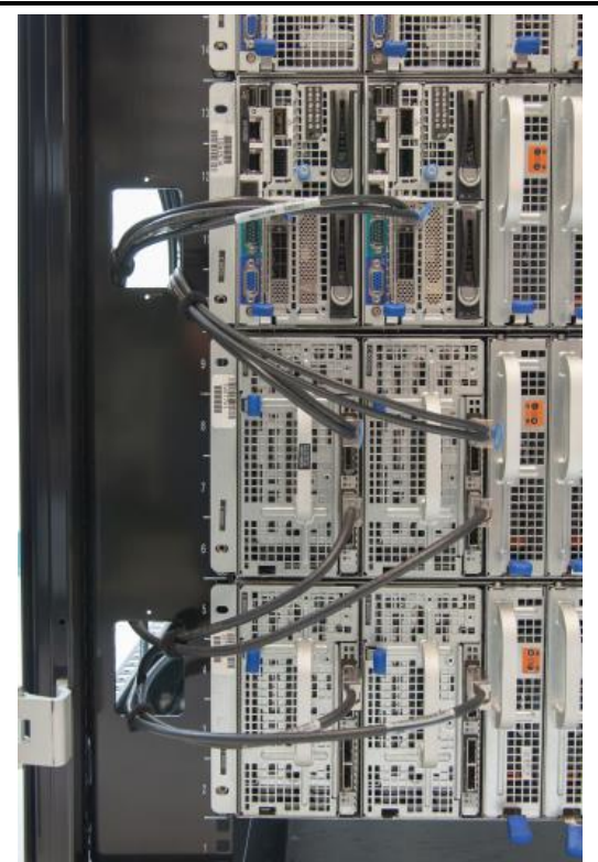
Figure 14: SAS cable installation.
