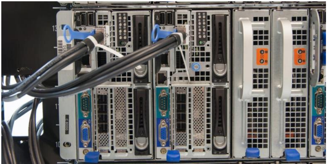
Figure 12: Ethernet cable installation with 40GbE connectors.
