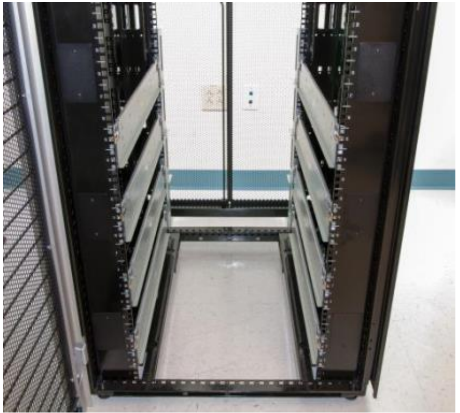
Figure 2: Rail and rack installation.
